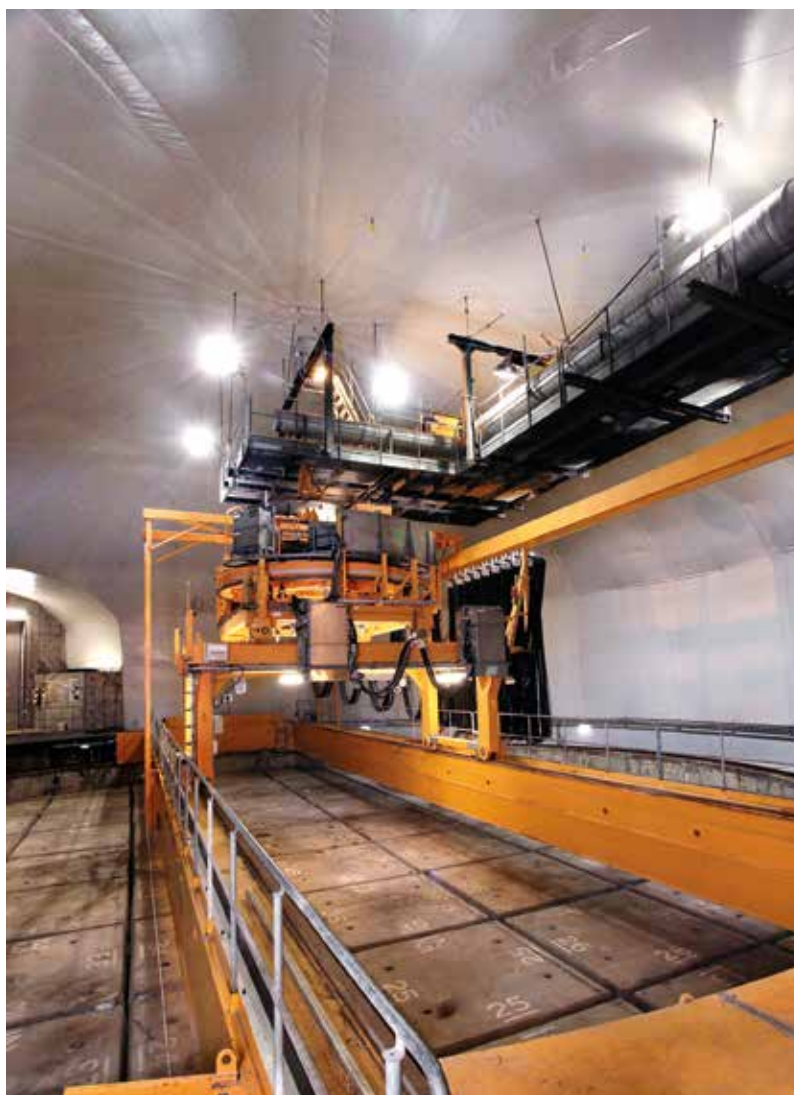
Figure A7: Photo from the top of the silo in SFR.
